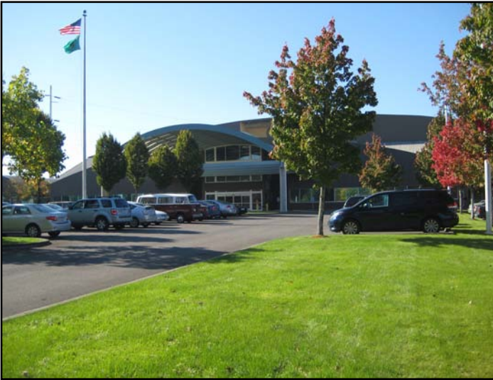
The Distribution Center is located in Seattle.
